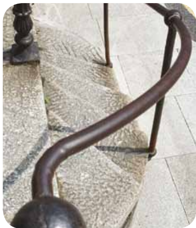
Granite steps - Penzance
